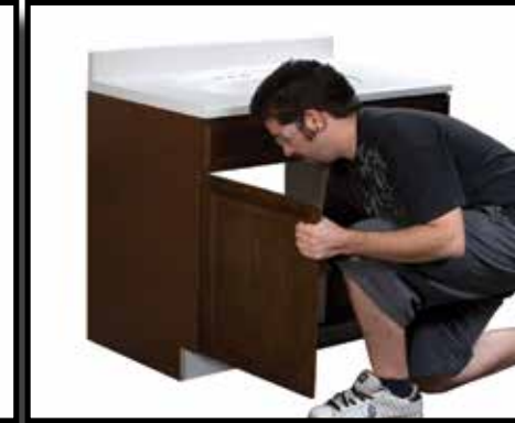
Step 2 ADA VANITY: Carefully remove doors and set aside for later use
