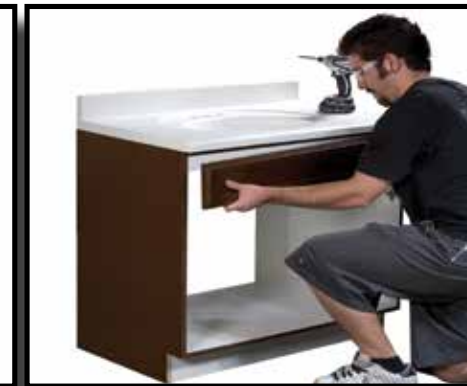
Step 4: Unscrew header from bracket with normal Phillips Head screwdriver
