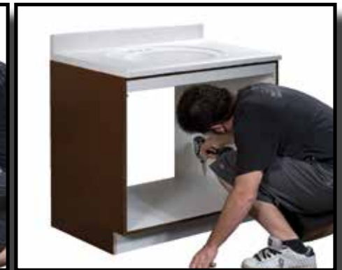
Step 5: Remove floor screws (4)
